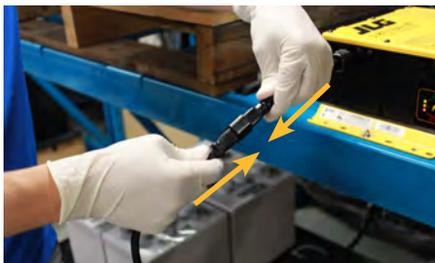
Figure 4: Reconnect AC power to the charger
